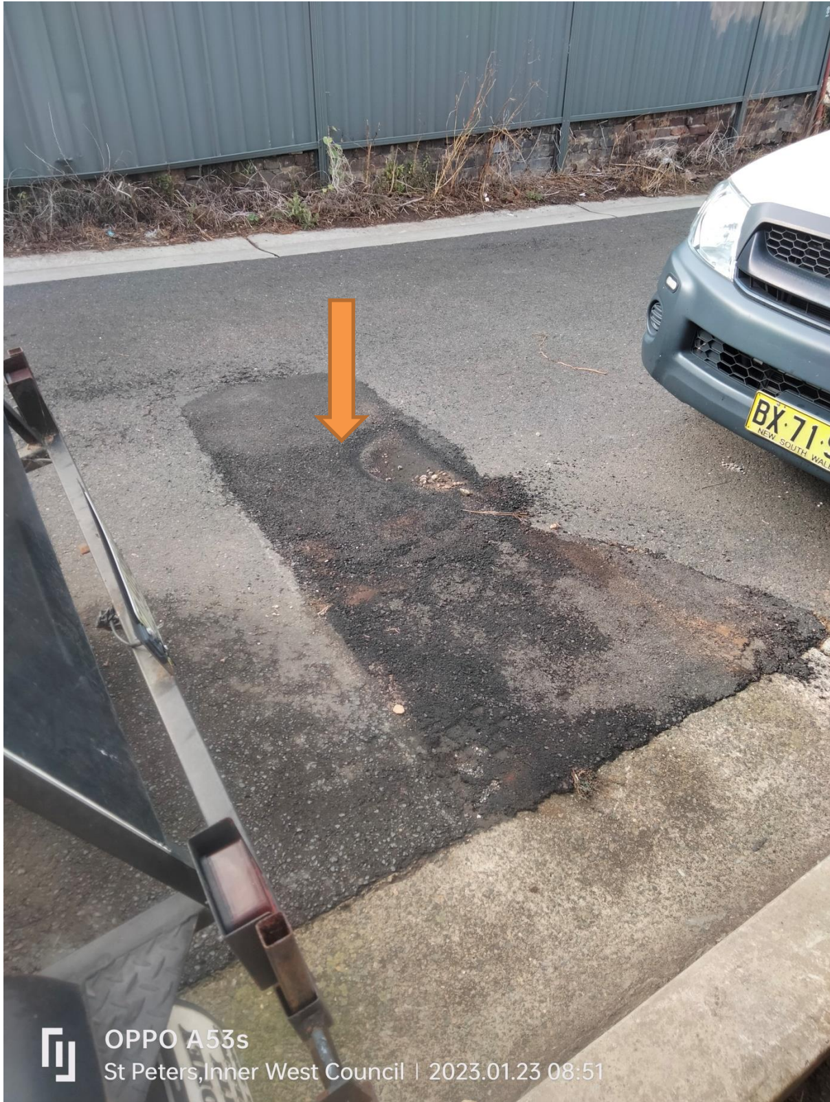
Figure 14 the rear road had filled in location with existing damage to the road behind number 118 where the garage is to be demolished and built.
