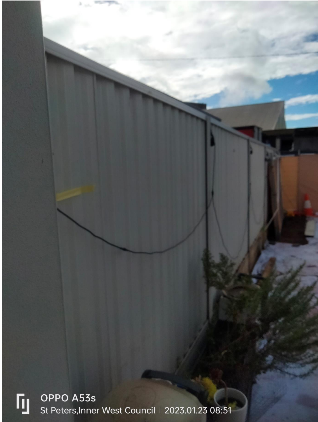
Figure 13 the dividing metal fence between 118 and 116 rear view.
