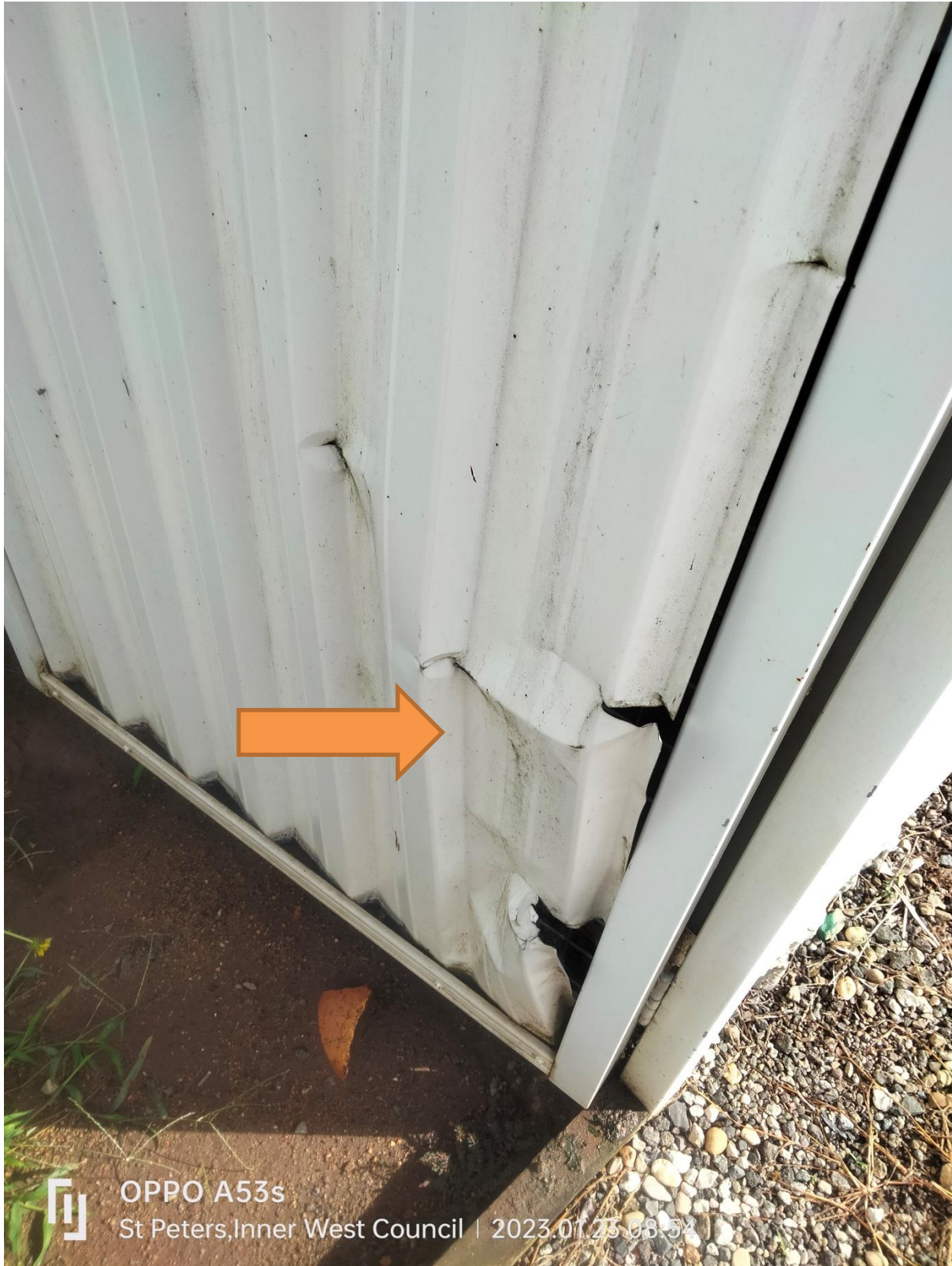
Figure 18 rear metal gate of 116 has metal gate damage observed.
