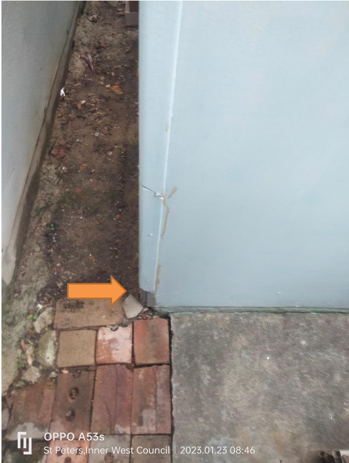
Figure 7 impact damage observed to the garage of number 120.
