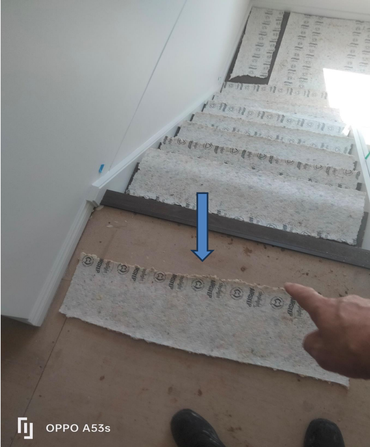
Figure 14 squeaking observed at the top of the landing, builder to investigate and rectify.
