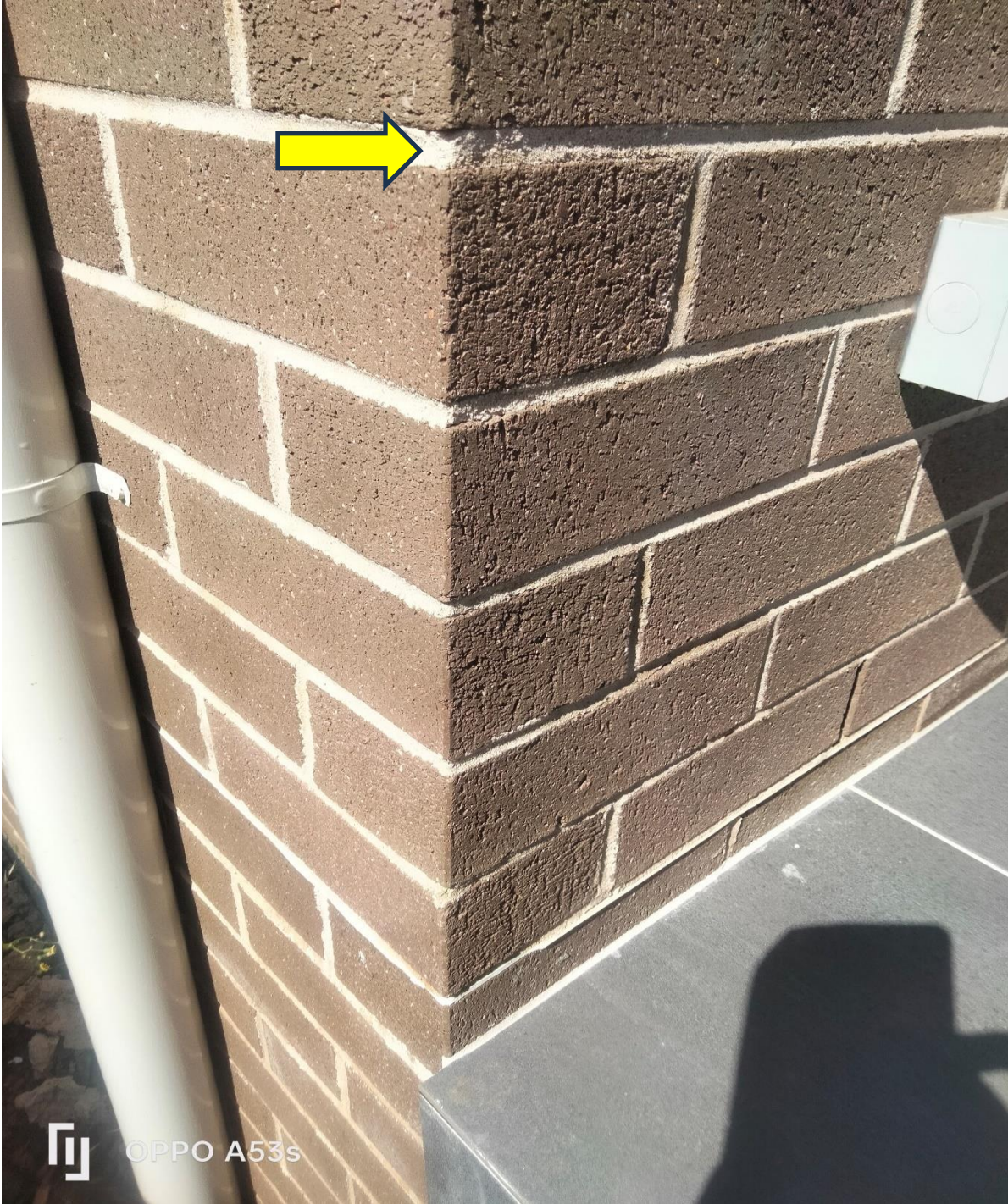
Figure 26 rear alfresco brick piers were observed as incomplete. This is non-compliant work.
