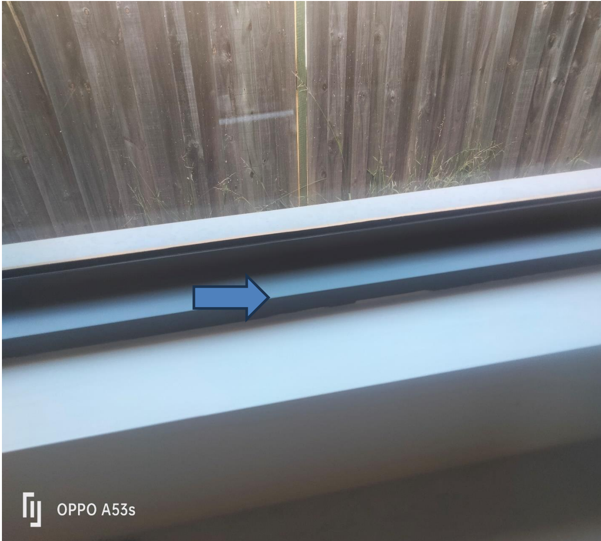
Figure 7 kitchen window was observed as having over painting and this requires completion to an acceptable standard, this is incomplete work. All windows should be inspected by the builder and corrected where applicable.
