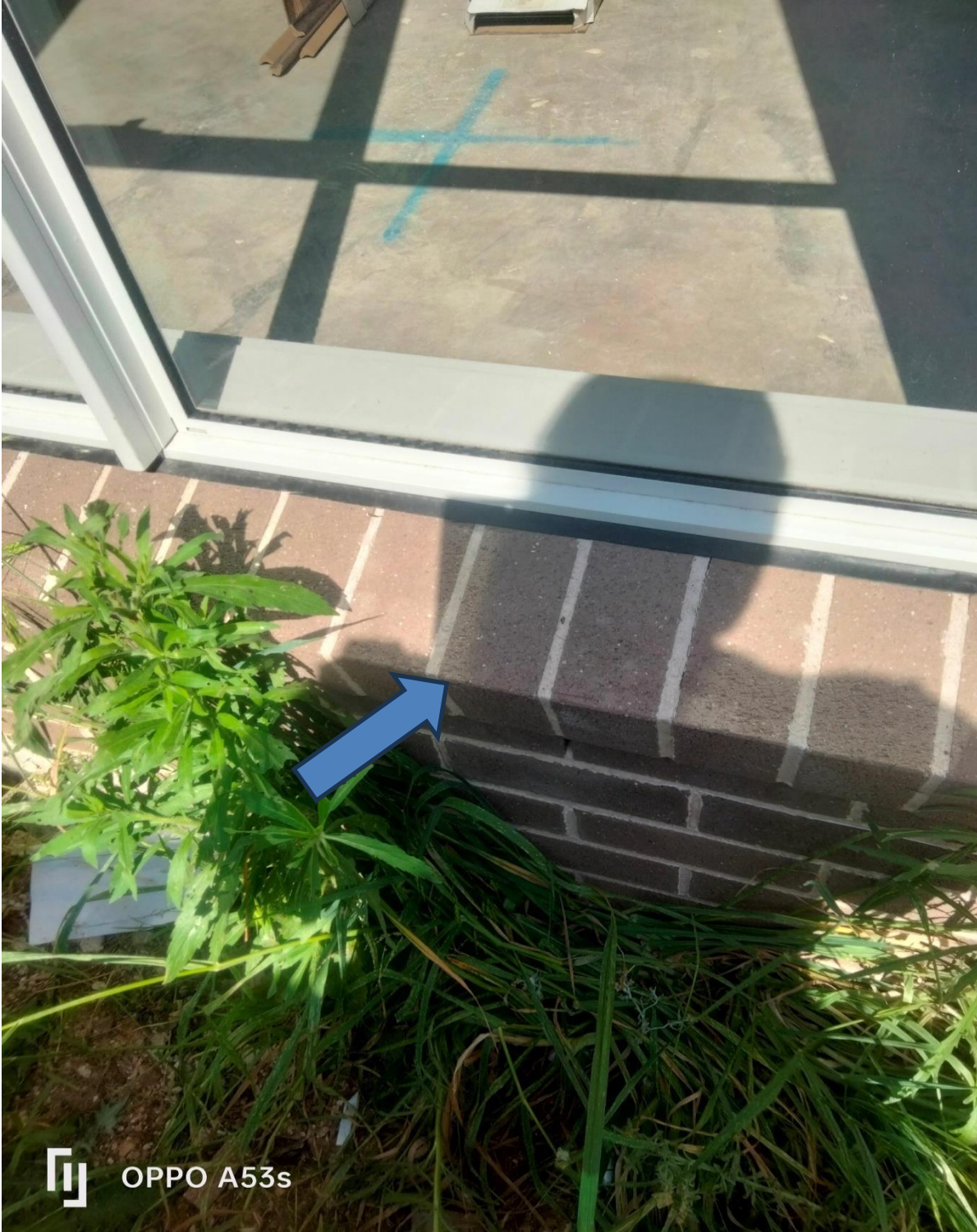
Figure 25mortar requires completion.
