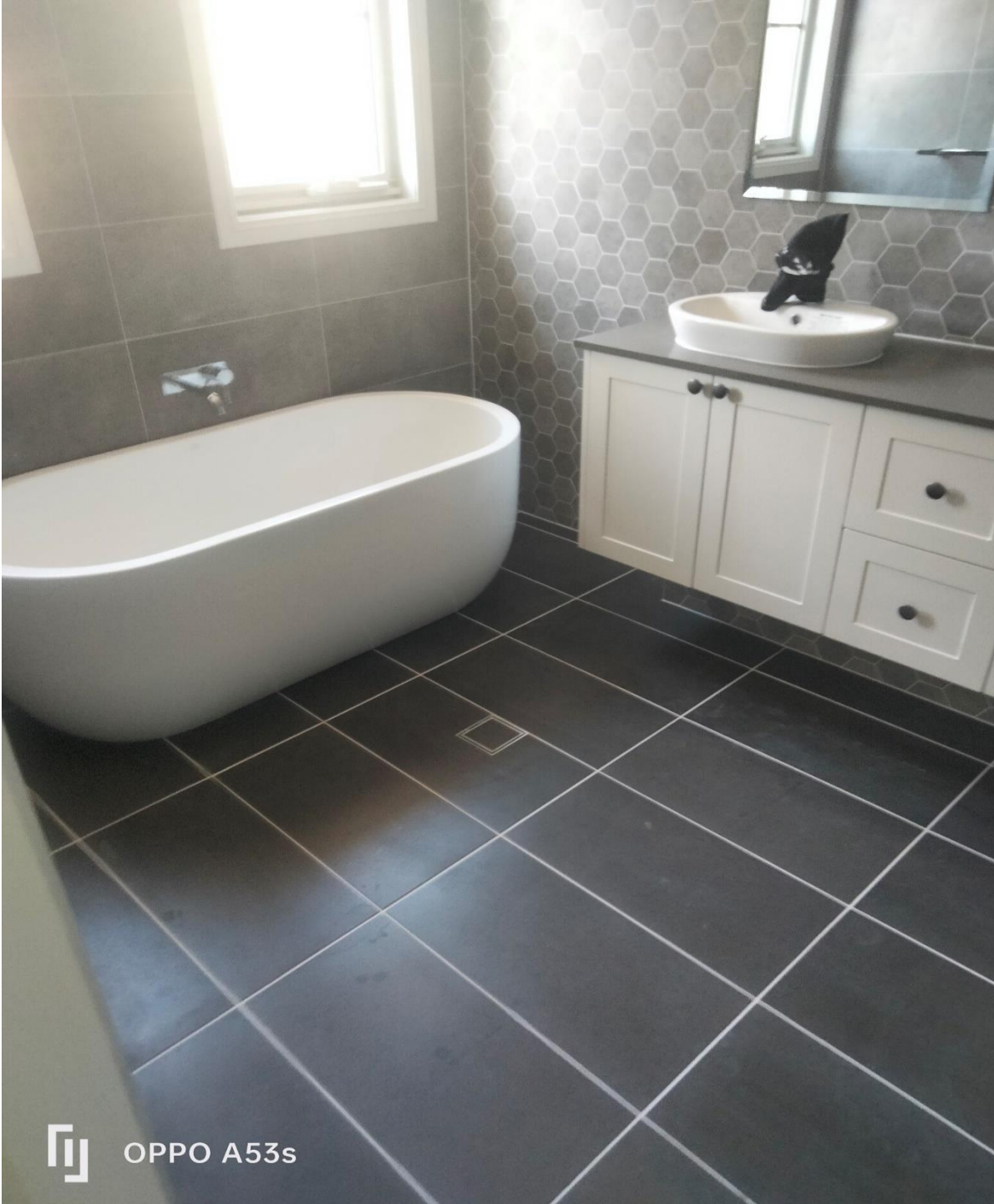
Figure 18 the bathrooms were inspected.
