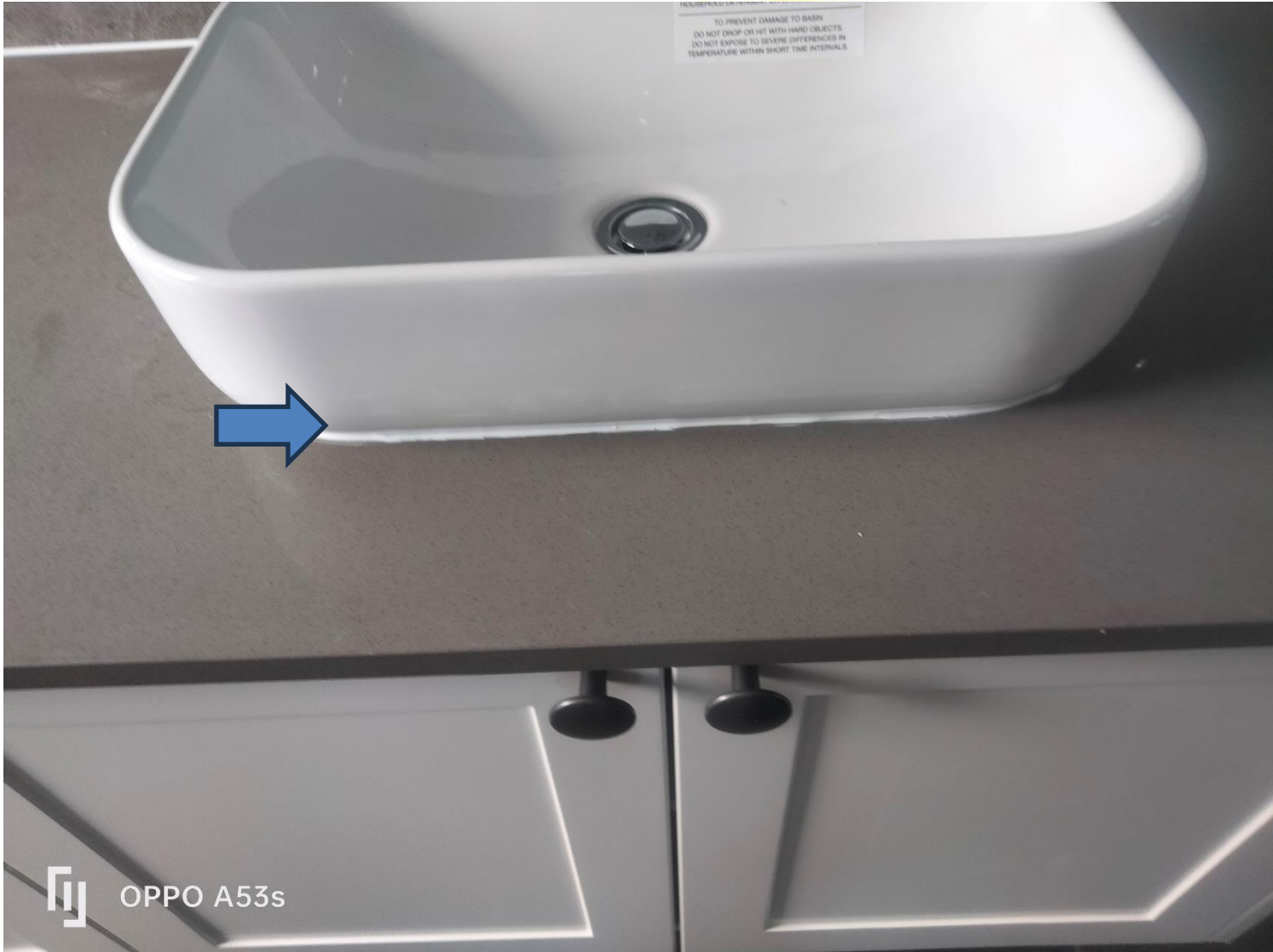
Figure 12 Rear ensuite vanity left hand side facing from the back has poor silicon application requiring completion.
