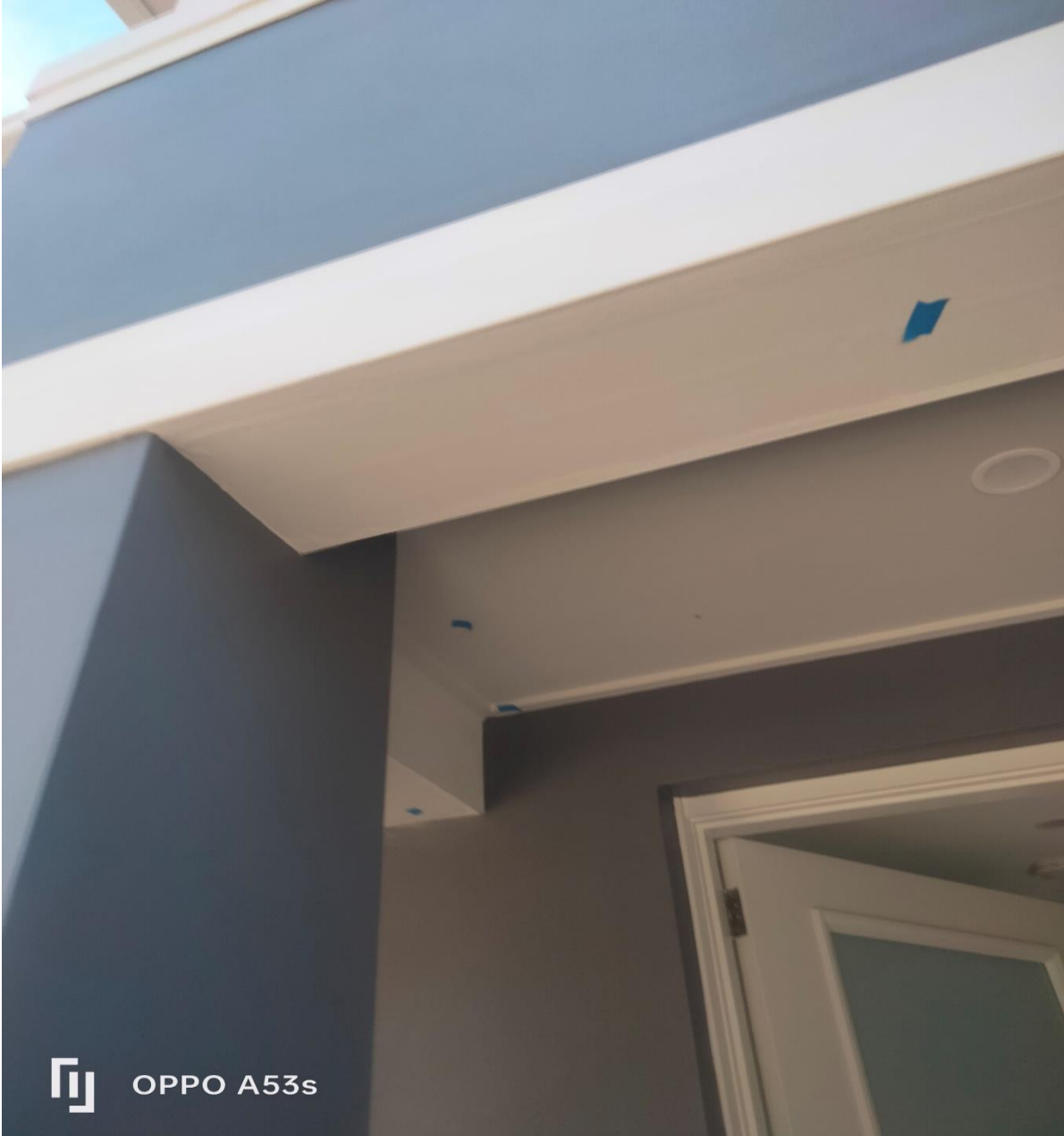
Figure 32 front entrance surrounds require final painting.
