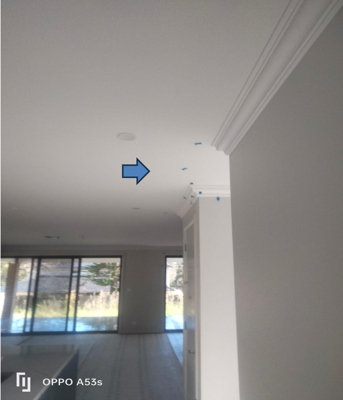
Figure 4 ground floor lower landing location.
